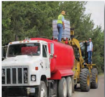
4) Mix one part Envirotac II to 12 parts water
