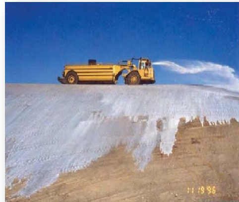
Envirotac II being applied.
