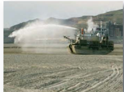
Tailing Pond Machines
