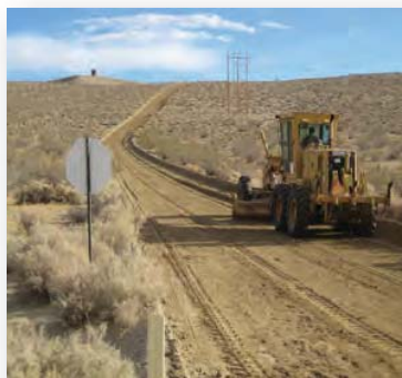
8) Blade soil at center to grade.
