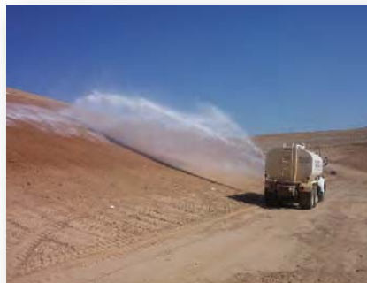
Slope Erosion Control
