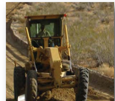
6) Wind roll soil to the center of the road
