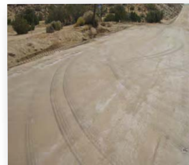
12) Finished road is hard as a rock!
