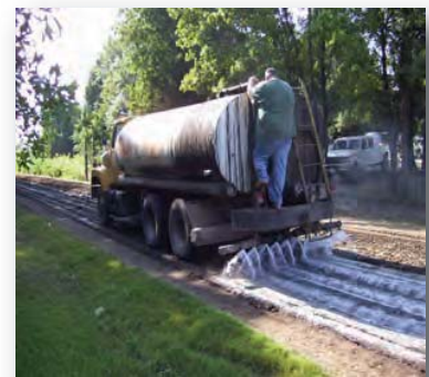
9) Apply one coat of Envirotac II
