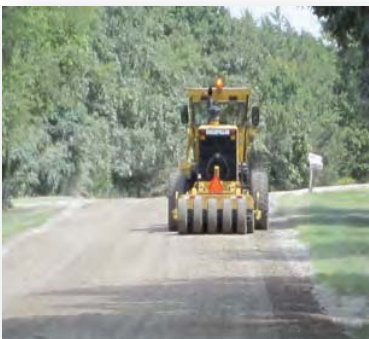
10) Roll area to 95% compaction
