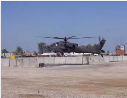
Helicopter Landing Pads
