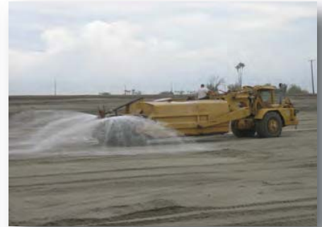
Construction Site Dust Control
