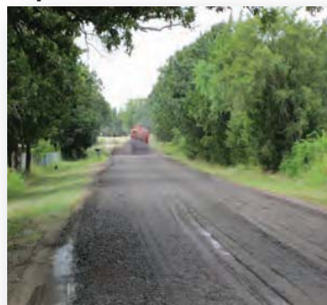
5) Apply Envirotac II solution to disturbed road
